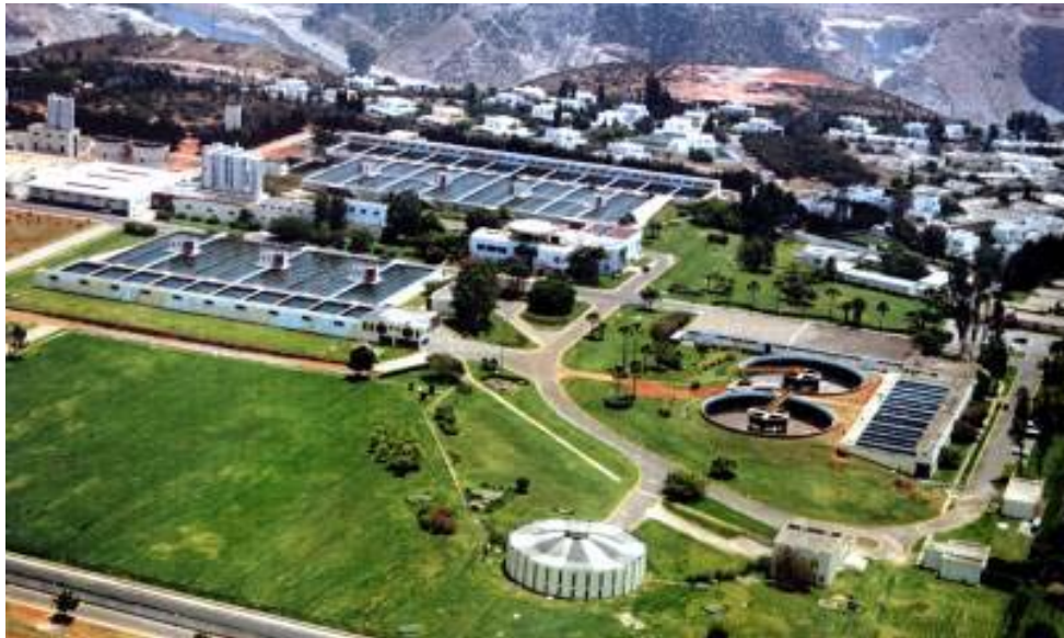
Bouregreg treatment plant (800 000 m 3 /d) ONEP- RABAT
